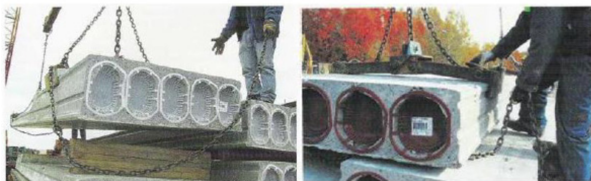
Figure No.5 Putting on and removal of safety chains
